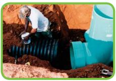
**STEP 3:** Install provided F-477 gasket for HDPE/PP corrugated pipe into last corrugation of the pipe. Lube the gasketed pipe and the inside of the drain basin bell.
